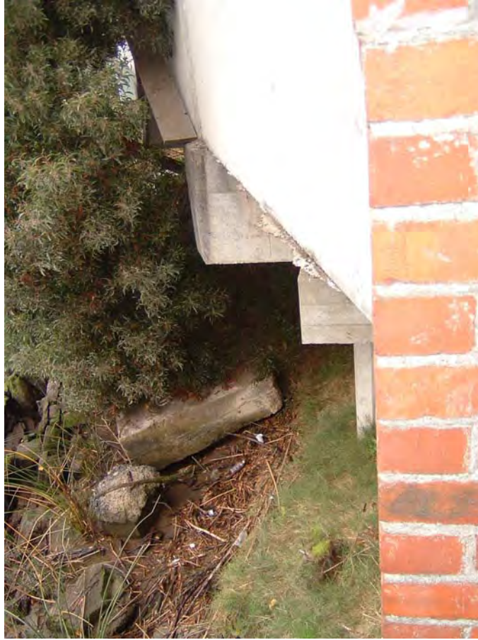
Photo 5. View of cantilevered portion of the historic Napa Mill building. The soldier pile wall will be 10 feet to the left of this building wall.
